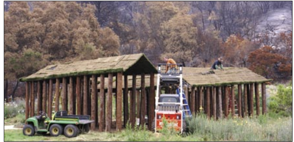
The construction of Labyrinth: Respite , by Herb Parker
