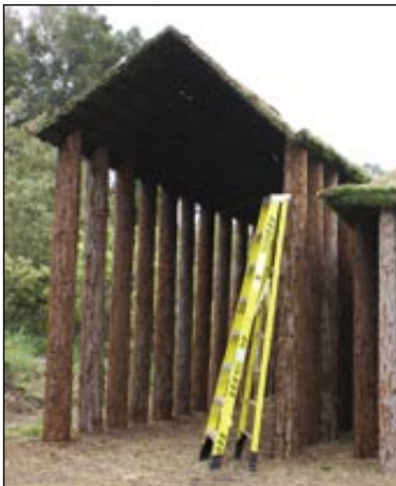
Labyrinth: Respite , redwood, sod, & rebar, by Herb Parker
